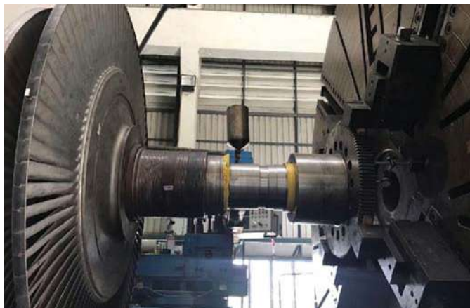
Fig. 3 • The turbine shaft mechanically prepared for welding.
