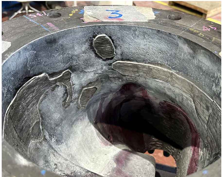
Fig. 5: Areas repaired by pulsed laser beam welding (© DSI-Thailand)
